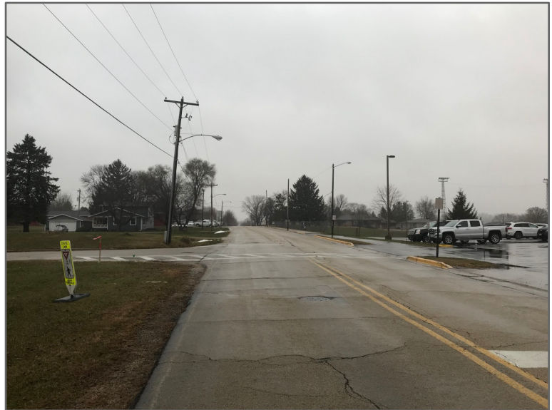
Figure 14. Sidewalk improvements are recommended for the west side of 2nd St, seen here.
